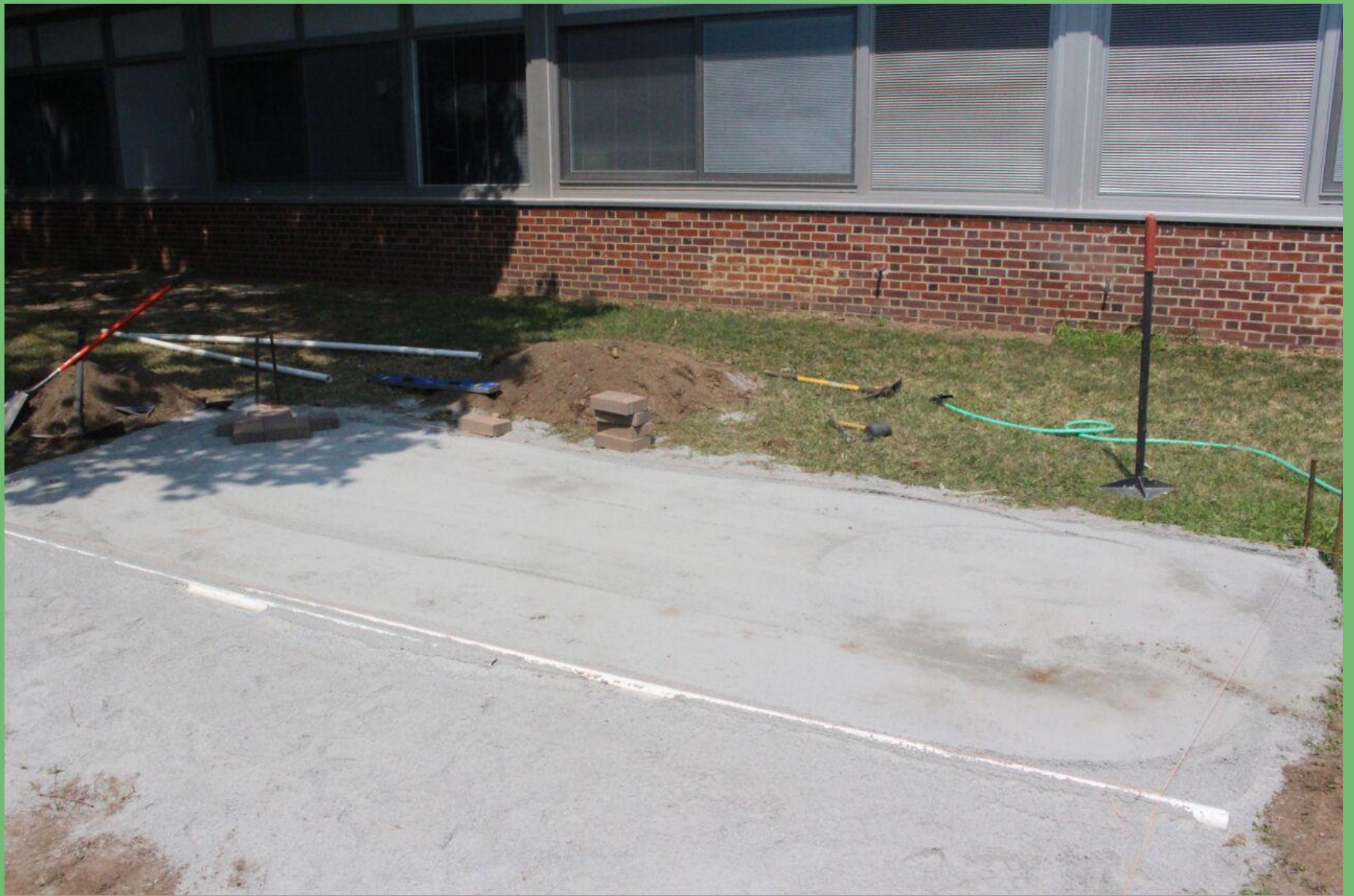
Preparing for the pavers....
