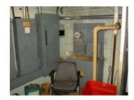
(6) distribution circuit breakers and one new Square "D" MDP-2 with (3) distribution circuit breakers. MDP-1 is protected with a 400A main circuit breaker (MCB). MDP-2 is protected with a 200A MCB. JCP&L is the utility company serving electrical power under account #100006467532. In August of 2007 the max demand was 67.4 kw/187A.
