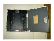
Newer computer panels have been installed to feed computer areas. A 225kVA "K" rated transformer was seen installed on the line side of the computer distribution panel (CDP) to mitigate harmonics.
