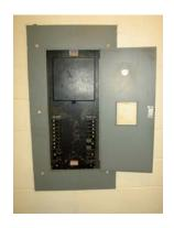
found to be loaded to circuit breaker capacity and lacking spares or spaces. Newer computer panels have been installed to feed computer areas.
