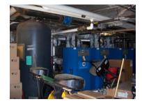
Gymnasium - The room is served by hot water heating & ventilating (H&V) units. The units are original to the building and appear to be in fair condition, though they have exceeded their expected operating lives.
