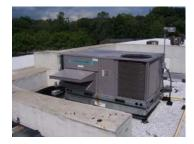
Media Center – The media center utilizes newer unit ventilators with hot water coils and remote condensing units to provide space cooling.
