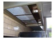
Multi-Purpose Rooms - The rooms are served by steam heating & ventilating (H&V) units. The units are original to the building and appear to be in fair condition, though they have exceeded their expected operating lives.
