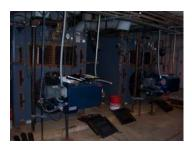
Auditorium - The room is served by steam heating & ventilating (H&V) units. The units are original to the building and appear to be in fair condition, though they have exceeded their expected operating lives.
