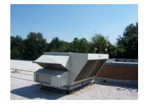
Media Center – The media center utilizes a newer gasfired, heating/cooling rooftop unit.
