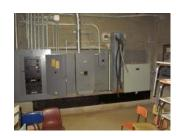
installed in the addition areas. A 225kVA "K" rated transformer was seen installed on the line side of the computer distribution panel (CDP) to mitigate harmonics.
