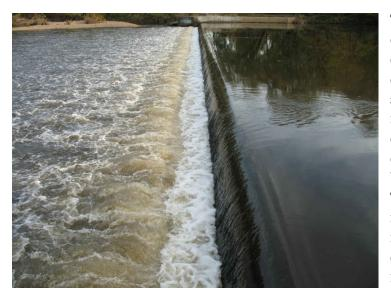
The Robert Street Dam was reconstructed in 1964 after the original dam at this location failed. The original dam had partially overturned, subsided, and was breached through numerous structural fissures that destabilized the structure, so that older structure was encased and buried beneath the reconstructed dam. The removal of Robert Street Dam is a major Raritan River watershed restoration priority because it poses one of the most substantial impediments to fish migration
